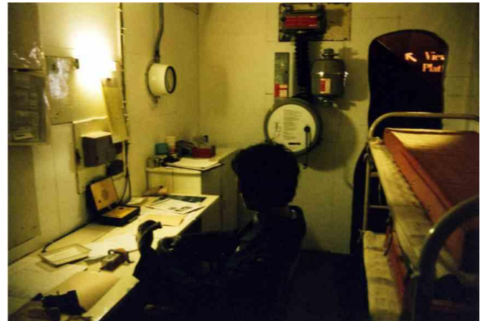
The recreated post at the Museum of Lancashire, the hole which Tony created through the 'concrete' wall can be seen to the right, as can the sign to the viewing platform. The Luwa air system is in the centre of the picture, its filter in the by-passed, i.e. the normal condition. The post office termination and test box are in front of the observer along with new style teletalk. Also the later type of FSM meter is shown buried in the desk, with a strap over it to prevent theft! (1994 – copyright Mike Norris)
