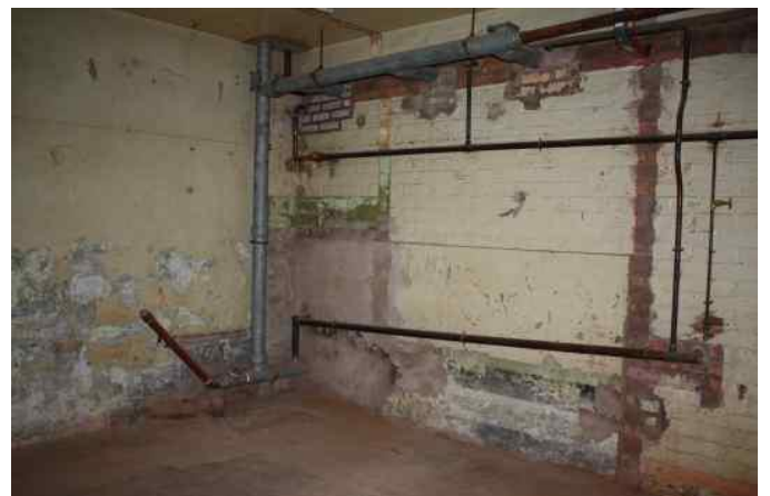
The former water tank room, in the control bunker. The pipe visible at 45 degrees is where the posts toilet room will eventually be located. (2009 – copyright Mike Norris)
